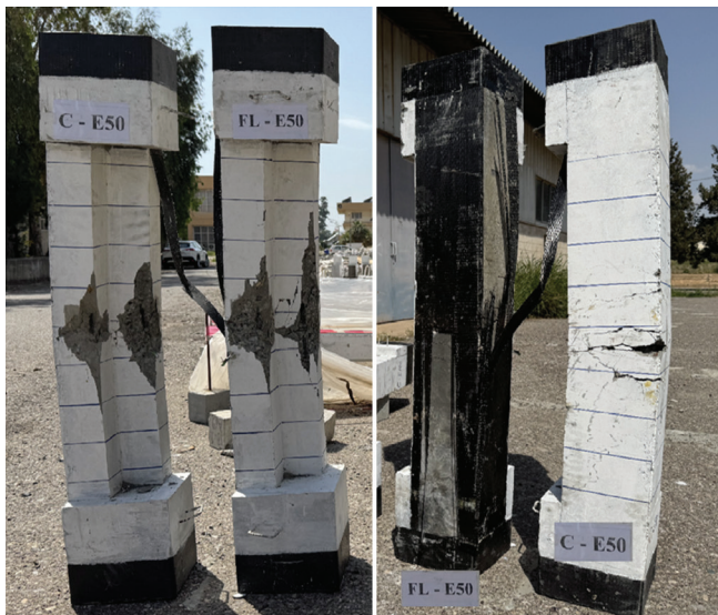
Fig. 7. Mode of failure and crack pattern of column specimens ( e_x = e_y = 50 mm).
