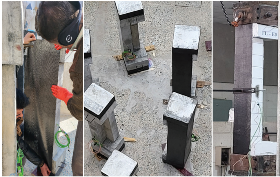
Fig. 4. Applying carbon fiber-reinforced polymer to flexural direction of columns.
